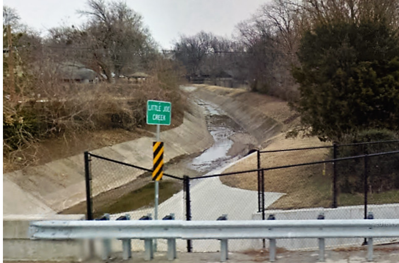
Little Joe Creek channel, looking east—upstream—from Hudson Ave.
