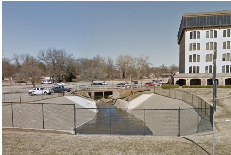
RLA #59 is about ¼-mile west of where the West Branch of Joe Creek emerges from underground and passes beneath Skelly Dr. and I-44.
