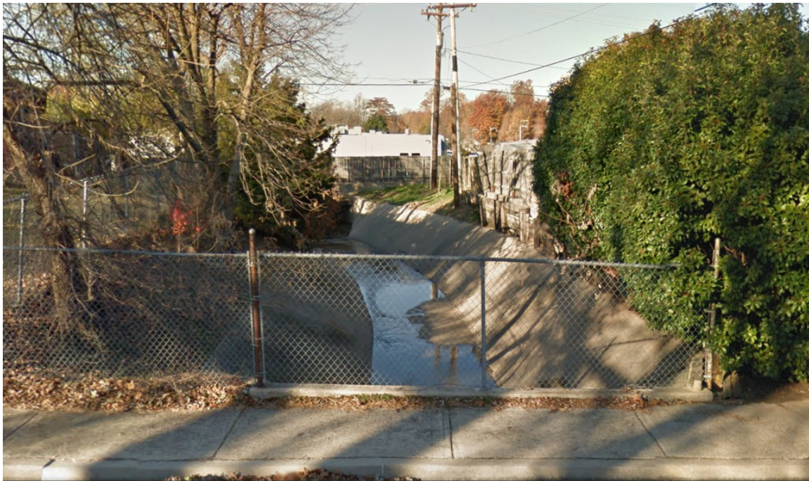
Little Joe Creek channel, looking west—downstream—from S. 67 th Pl. E.
