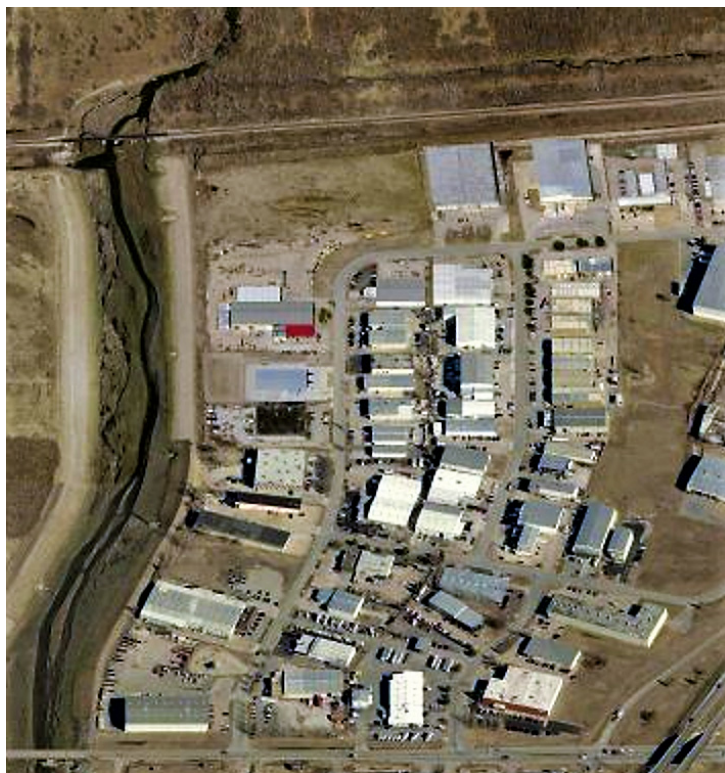
RLA #50 is built on what was once the meandering course of Mingo Creek. The channel was relocated about 400 feet to the west and the land filled to accommodate the new industrial park.
