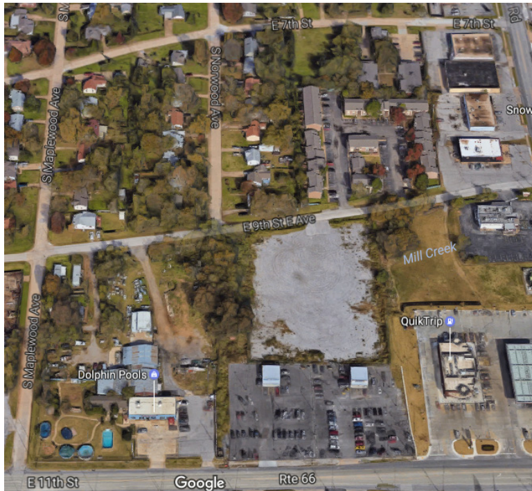
RLA #44. Mill Creek is carried in storm sewers from E. 11 th St. northeast to E. 7 th St. and Sheridan Rd.
