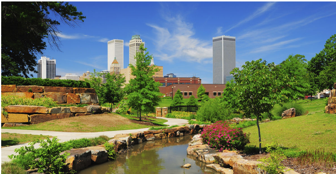
Centennial Park detention facility on Elm Creek near downtown Tulsa
