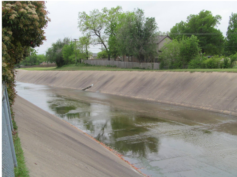
Joe Creek channelization near E. 57 th St. and Birmingham Ave.
