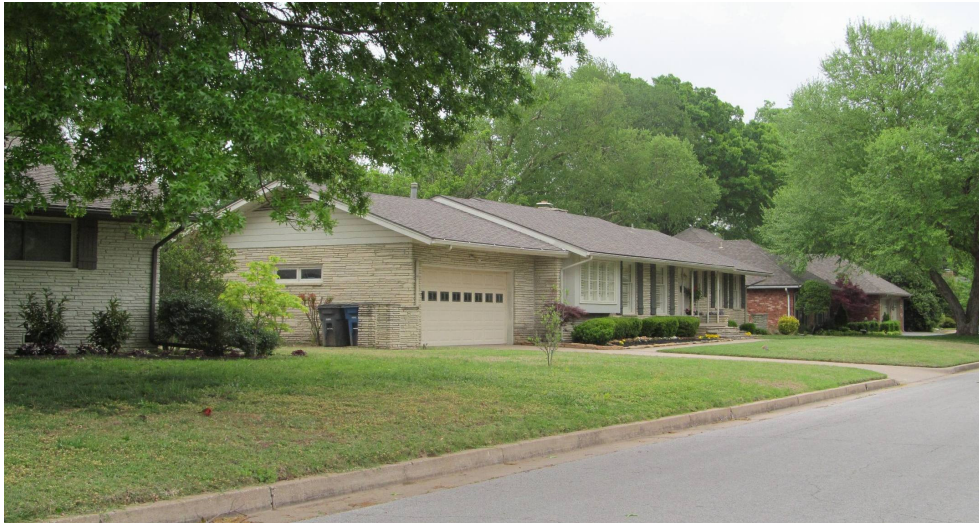
Since the completion of channel improvements along Joe Creek in the 1980's, the causes of flooding have been largely due to the level terrain, surface drainage issues, and slab-on-grade foundations.
