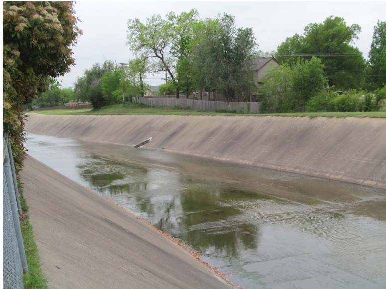
Joe Creek channelization near E. 57 th Pl. and Birmingham Ave.
