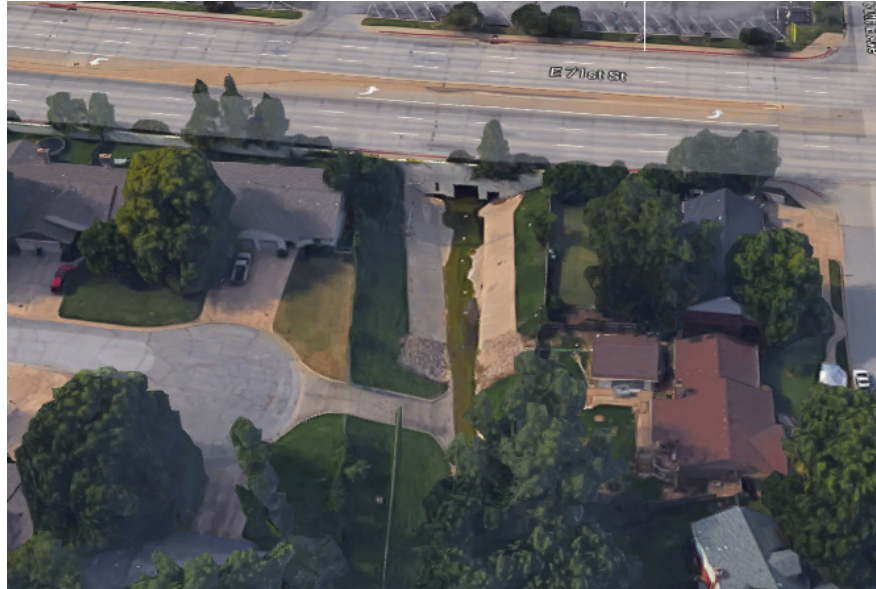
Little Haikey Creek emerges from storm sewers into an open channel on the south side of E. 71 st St.
