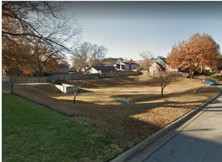
A small neighborhood detention facility was built immediately to the north of RLA #19 to prevent overland flow flooding.
