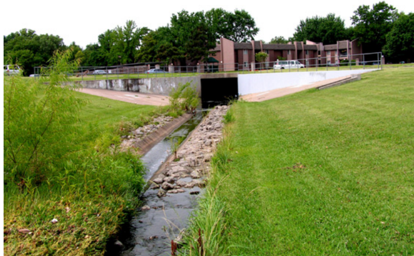
Little Joe Creek, looking west (downstream) towards RLA #17 from Yale Ave.
