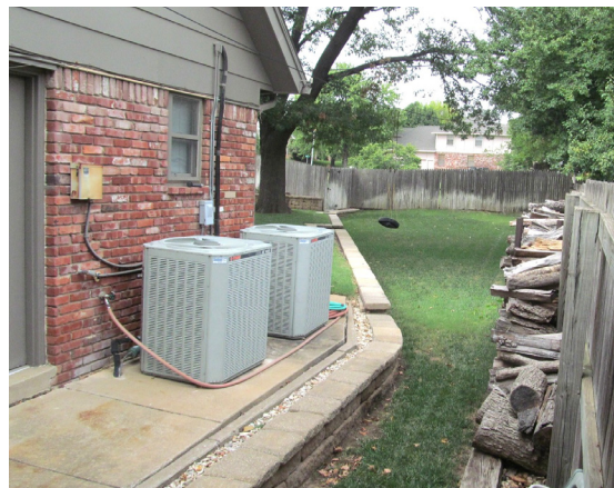
This platform and wall protect the home and air conditioning equipment from shallow flooding.
