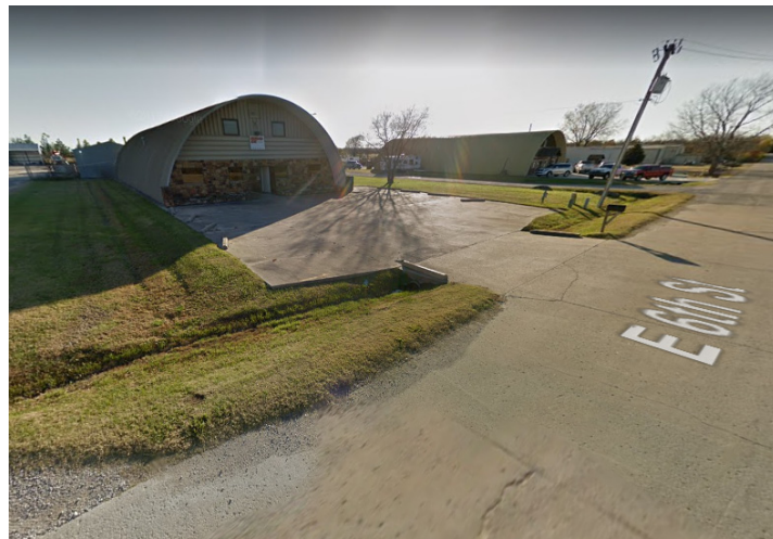
RLA #4 has shallow bar ditches in gently sloping terrain.
