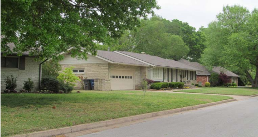
Since the completion of channel improvements along Joe Creek in the 1980's, the causes of flooding have been largely due to the level terrain, surface drainage issues, and slab-on-grade foundations.
