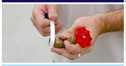
Prepare the threaded side of the <sup>3</sup>/<sub>4</sub>" faucet by wrapping it tightly with Teflon tape (make four or five rotations until all the threads are covered) or apply a thin bead of silicone caulk around the threads.
