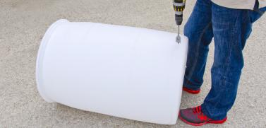
Use a 6" hole saw to cut a round 6" hole in the lid of your barrel.
