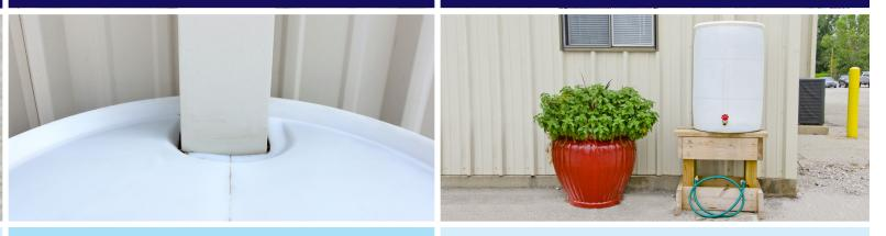
Cut your downspout about 4" above the top of the barrel, add the elbow from the bottom of the downspout and insert it into the freshly cut gutter downspout.
