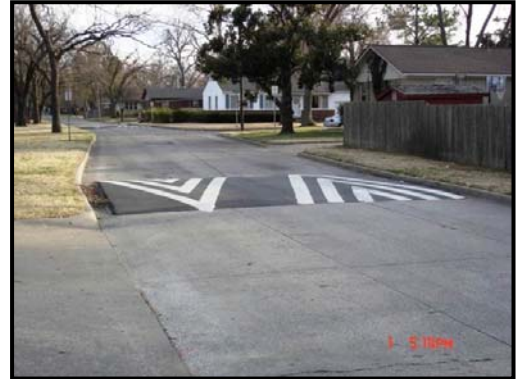
Figure 1: 22-Foot Speed Hump
