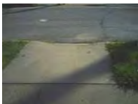
Ramp 4D Corner 4
