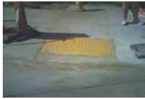
Ramp 4B Corner 4
